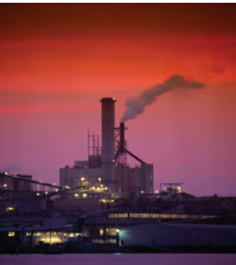
Sample and Instrumentation Filtration
