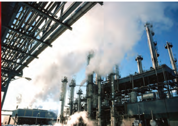
Instrumentation and Automated Pneumatic Controls
